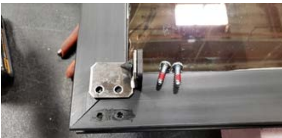
5. Picture of new door stop and screws
